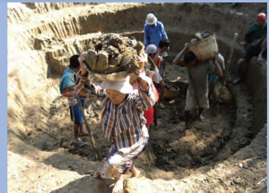
Brunnenbau in Kanazogo
